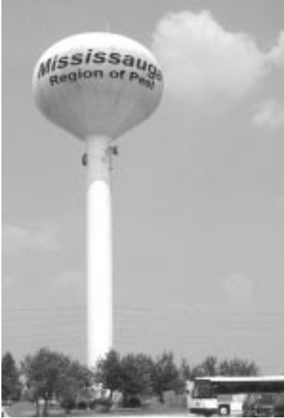
Our Water Tower gets a new look with the City and Region name.
